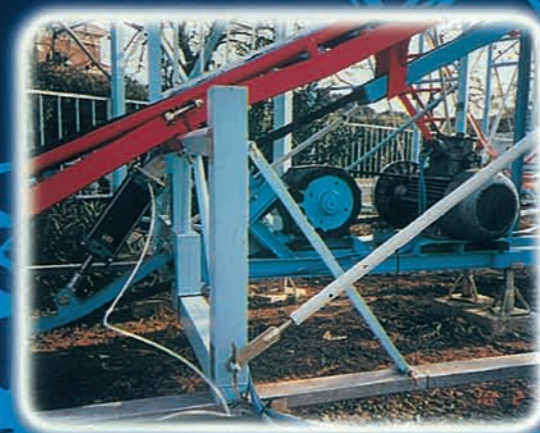
Drive motor located on the ground
